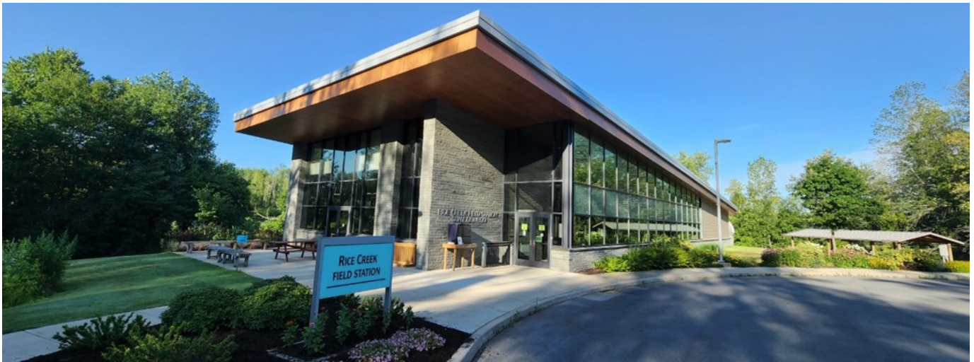
The LEED Gold research and education facility at Rice Creek Field Station, Oswego, NY.
